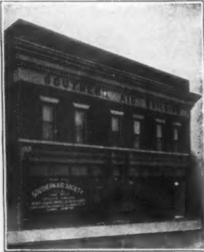
Society's Building, Danville, Va.
